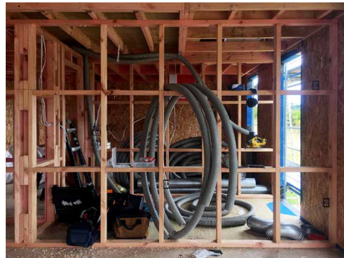
70mm flexible ducts for a balanced mechanical ventilation system - mid-install
